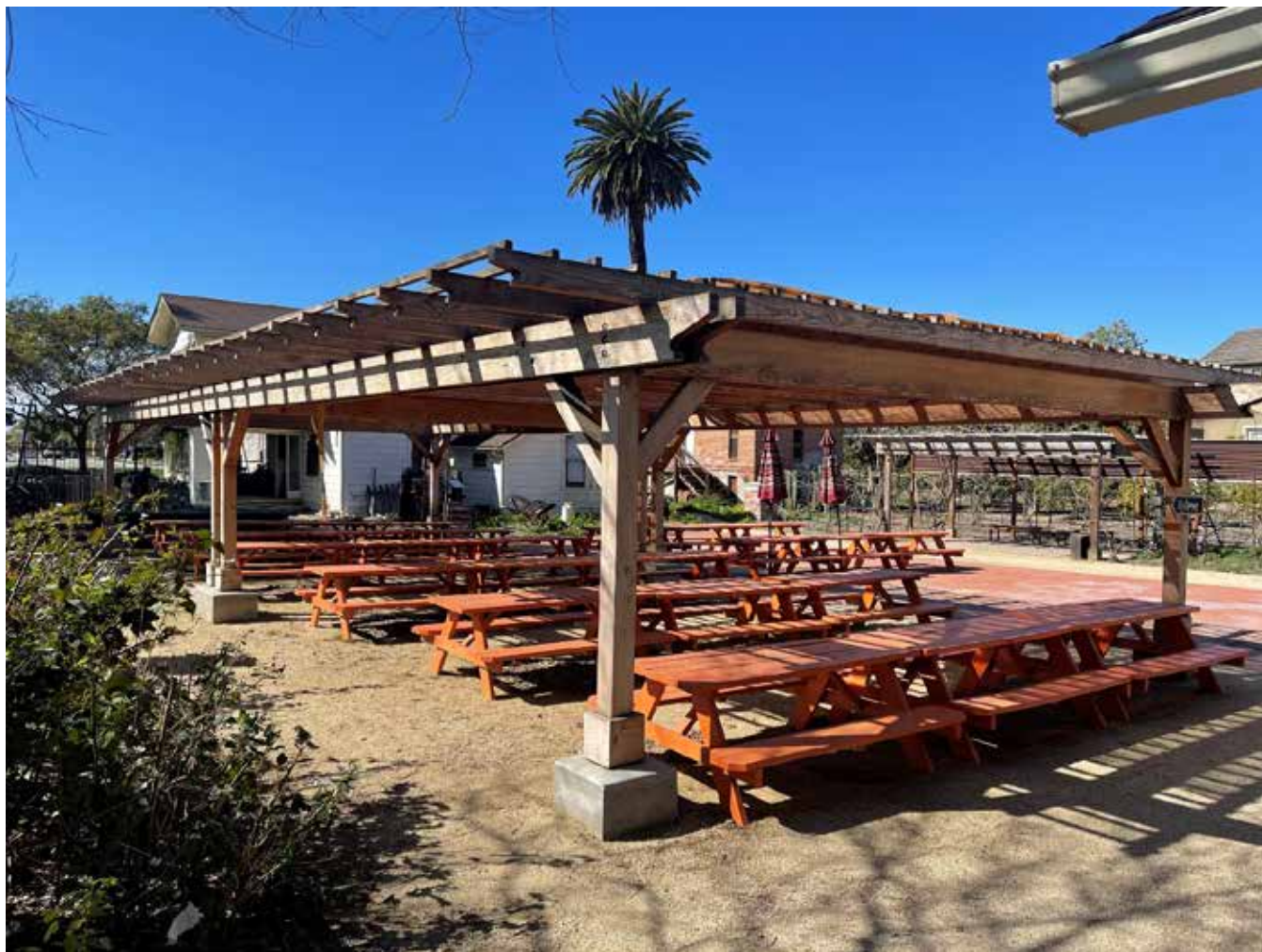
Figure 18 Noncontributing Pavilion (South East Elevation).
