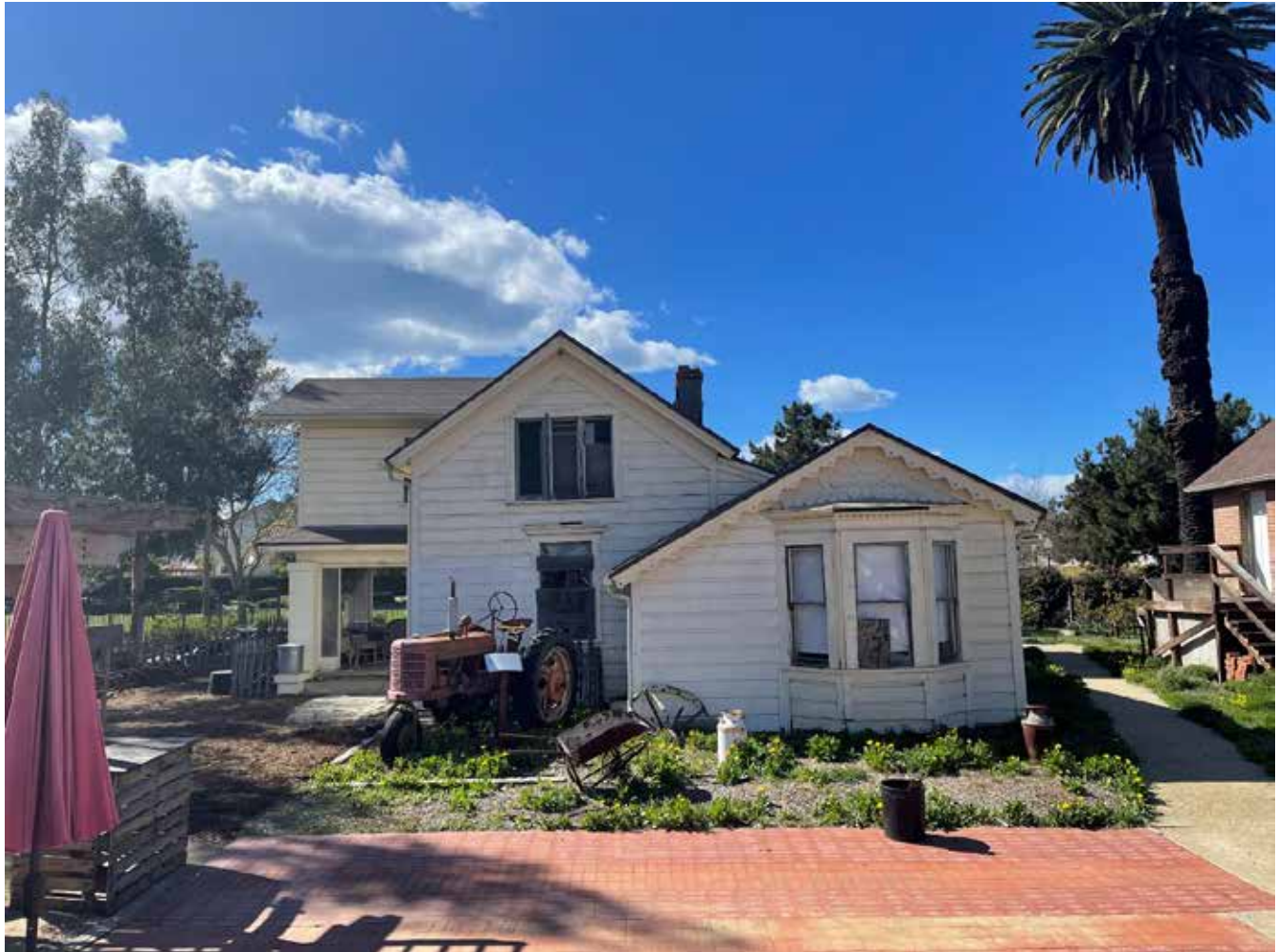
Figure 4 California_Ventura_Maulhardt, Gottfried Farm_0001 Contributing 1872 Farmhouse. (East Elevation).
