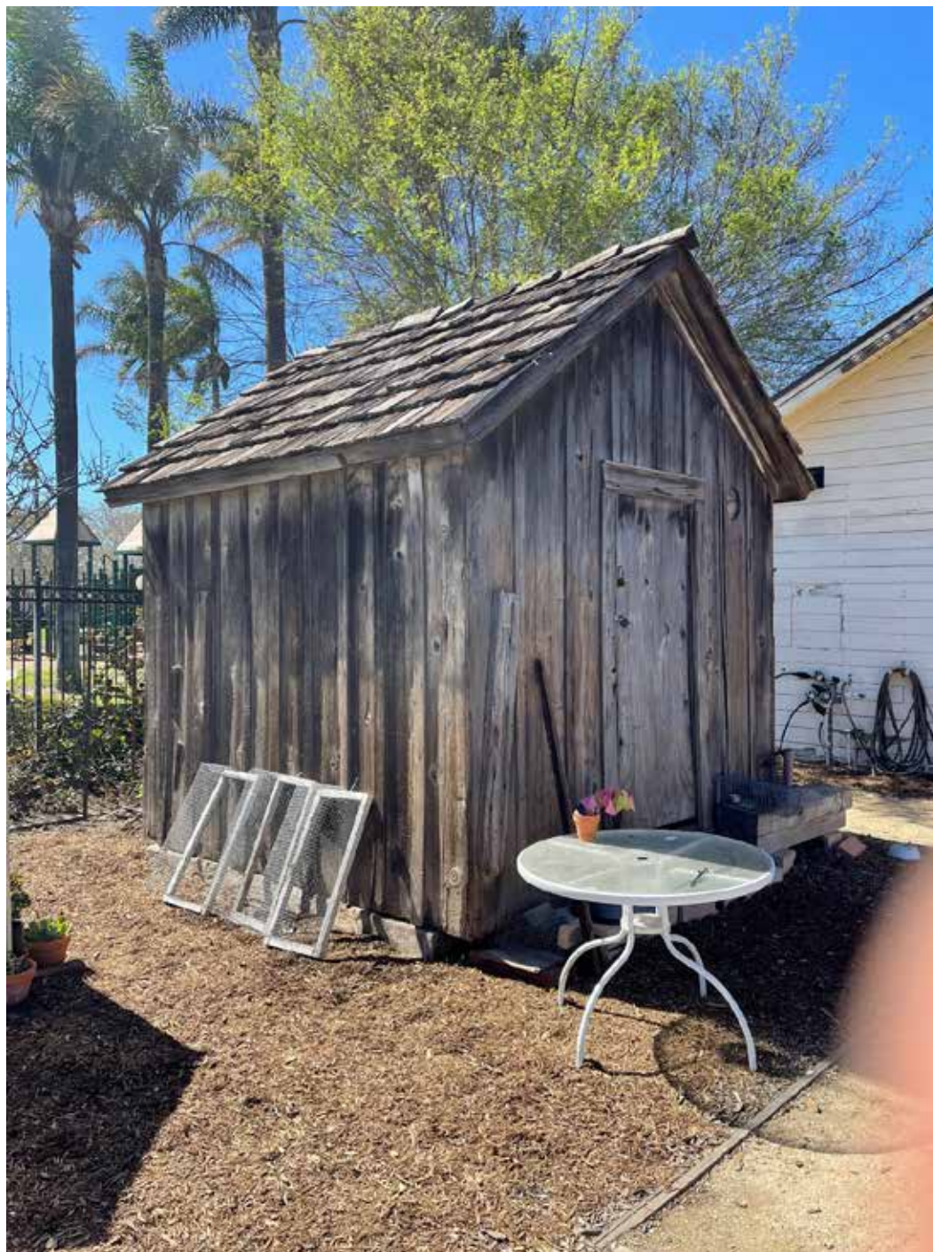
Figure 19 Noncontributing Bathhouse. (North East Elevation).
